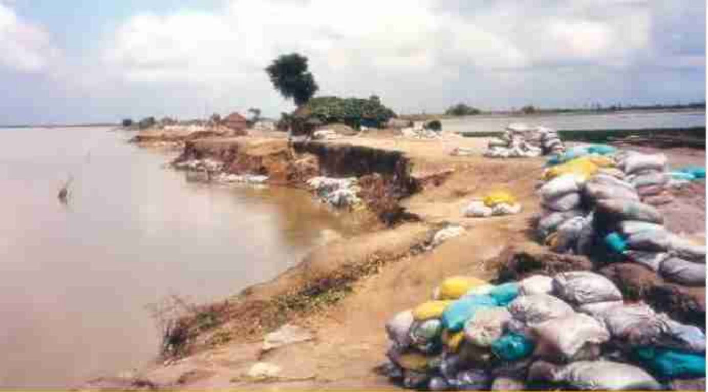
The embankments along the Kosi have led to drainage congestion and imparted, at some places, a false sense of security
